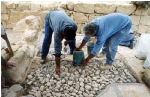
Bedding for a lime floor surrounding a mosaic
