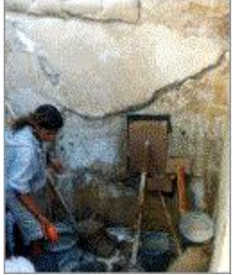
Supporting of lime plaster panels during consolidation
