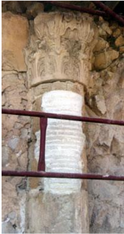
Filling of voids in columns with cast stone slabs
