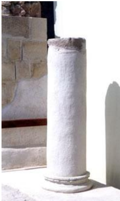
Cast, plastered column and base
