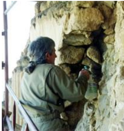
Filling "voids" in wall-core mortar.
