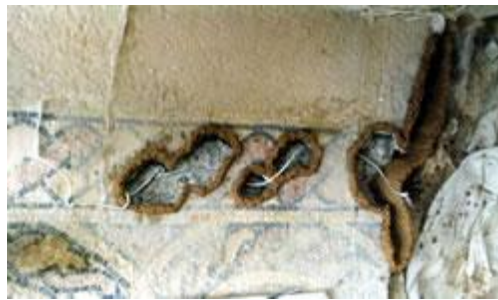
Injecting and filling of voids under the mosaic
