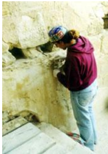
Conservation of fragile lime wall plasters
