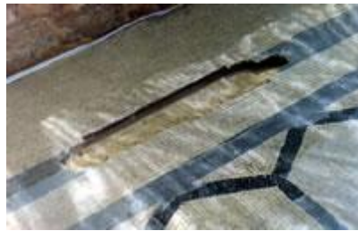
Mosaic floor during careful conservation treatment.
