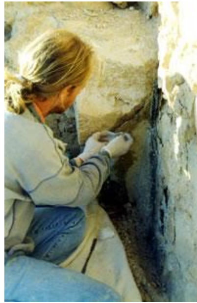
Filling of borders and cracks.
