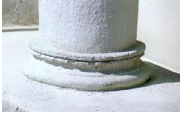
Detail of cast base before final coat.
