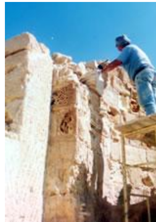
Bedding mortar in vault reconstruction.
