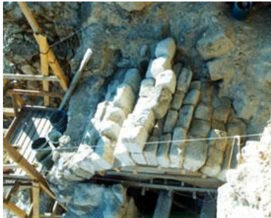
Bedding mortar in vault reconstruction.
