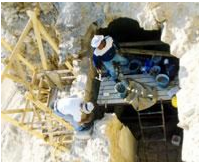
Reconstruction of a vault of a Bath-House on the edge of a 400 metre abyss
