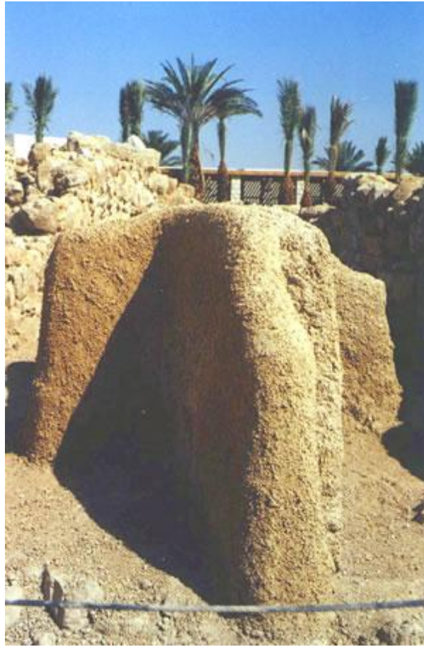
Retouching mud bricks, NHL 2/mud replastering and sacrificial protection layers
