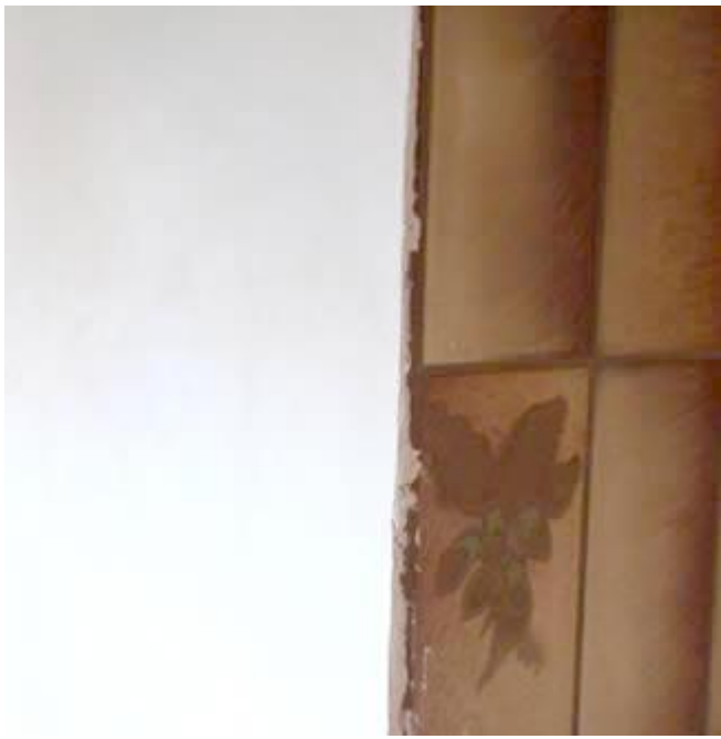
Plastering directly on tiles
