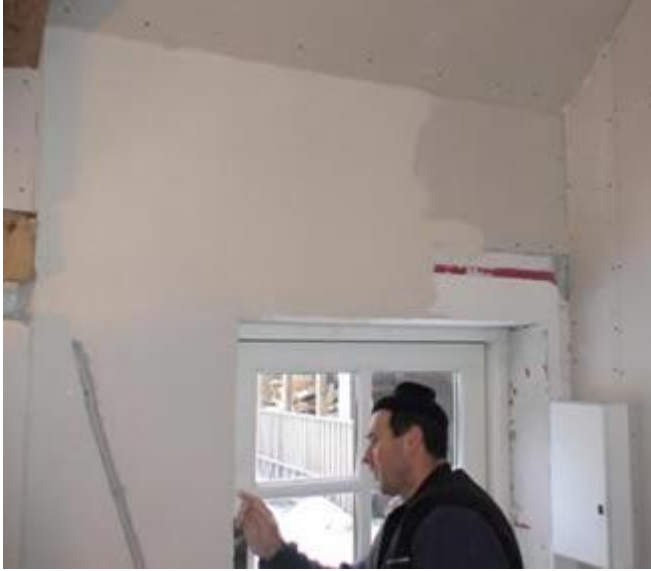
Applying Prependuit on different backgrounds (plasterboards+smooth cement+timber board)
