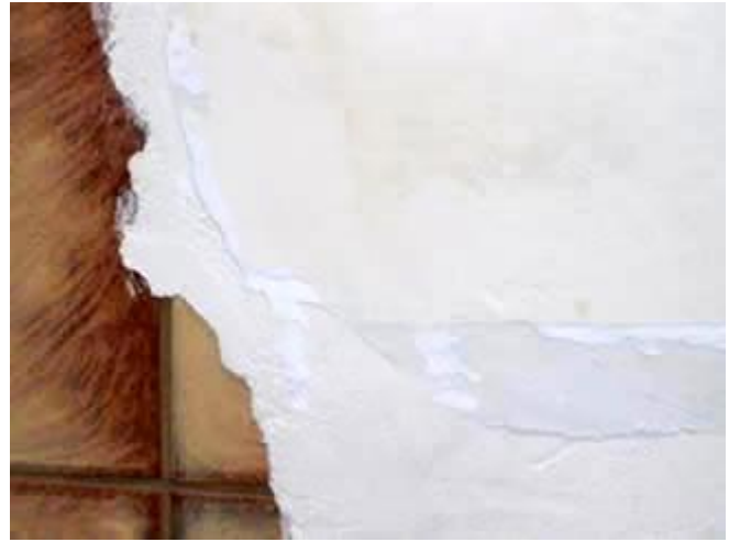
Smooth Plaster on tiles: 1st coat Prependuit, 2nd coat, Colour chausable F smooth finish with Col. Chausable EF.
