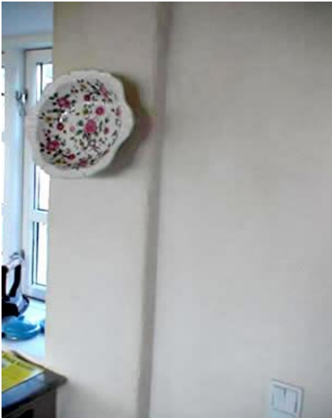
Chase area, finished
